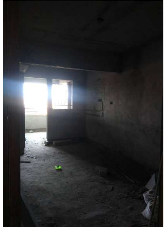
Figures. 4.6 Pictures of ongoing construction
