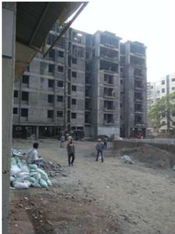
Figure. 4.7 View of Loknagari under construction building
