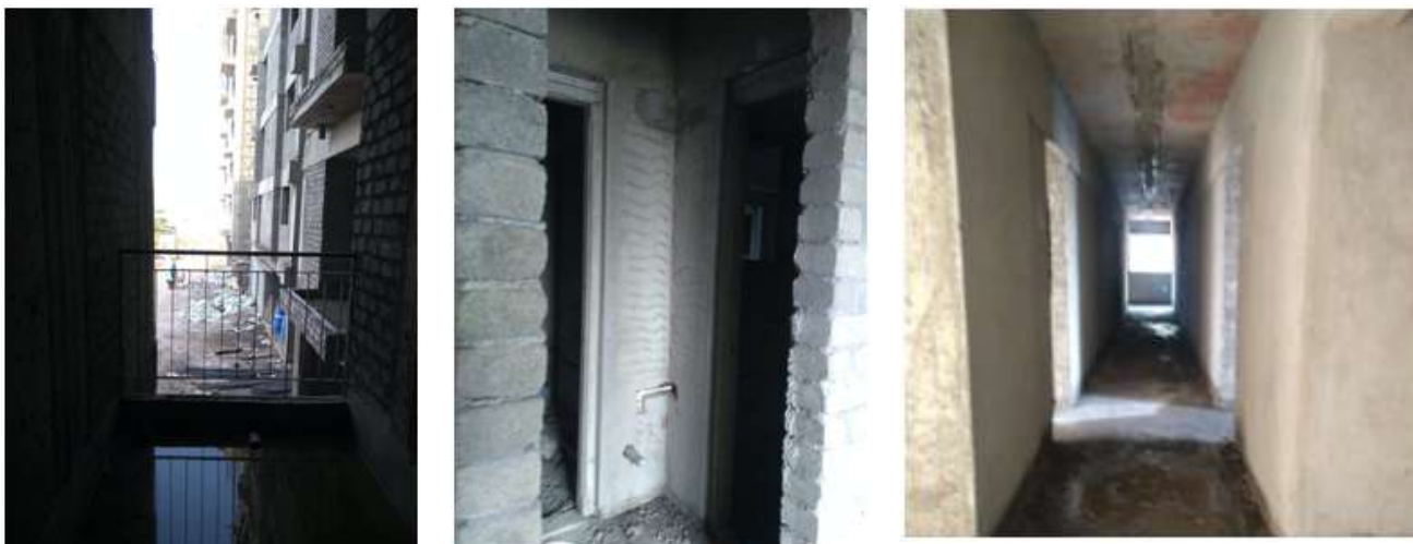
Figure. 4.9 View of Loknagari under construction building
