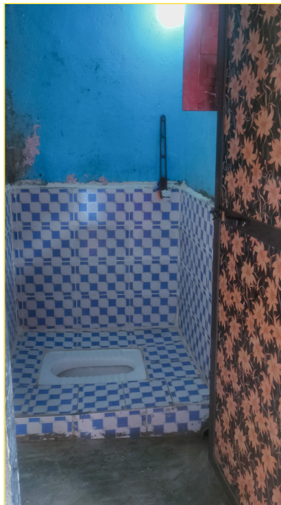
Kamble family's completed home toilet
