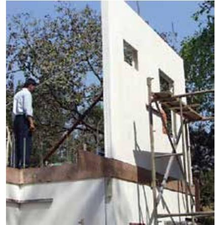
Construction of a model house using rapid wall technology in India
