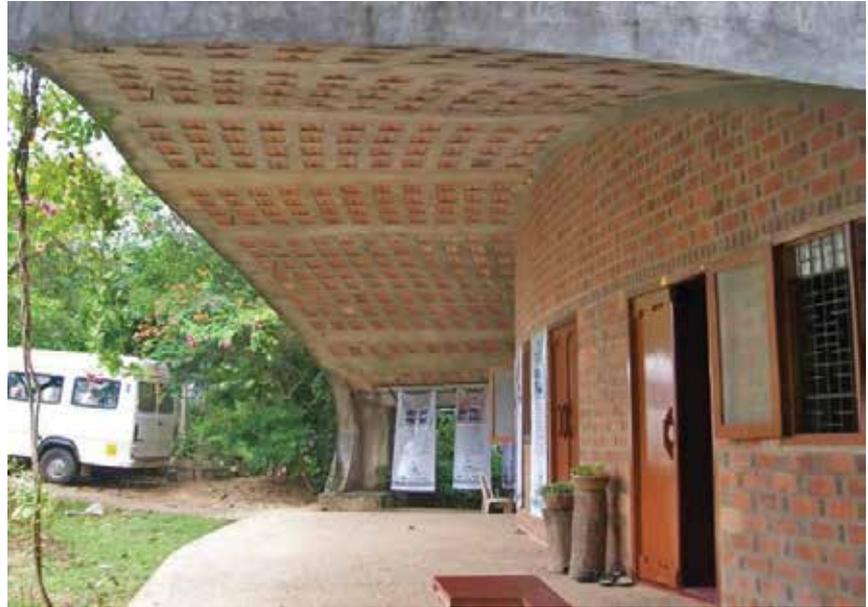
Picture showing a building at Laurie Baker Center, Trivandrum. Roof constructed using filler slab technique.
