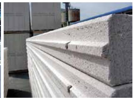
Interlocking edge of AAC wall panel
