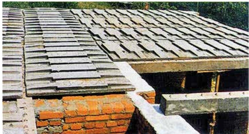
Roofing detail- Laying of precast RCC planks over RCC joists
