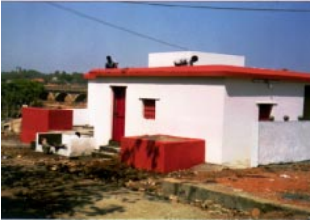
The new block: that's the caretaker's room in front
